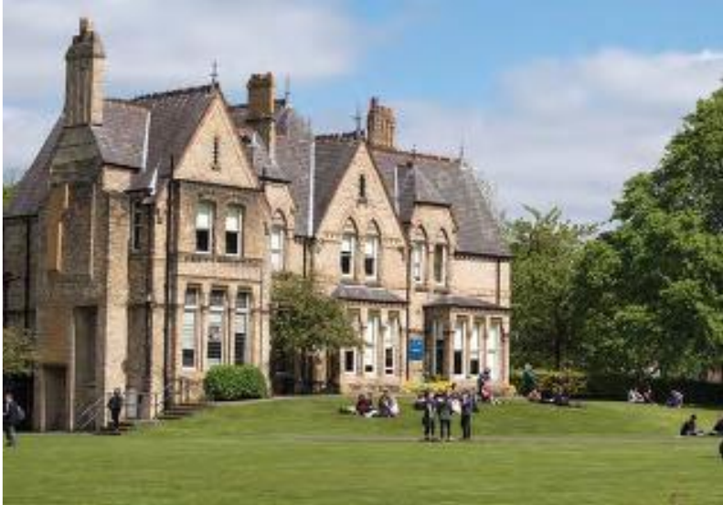
View looking north east towards Maryland across the open space in the foreground
